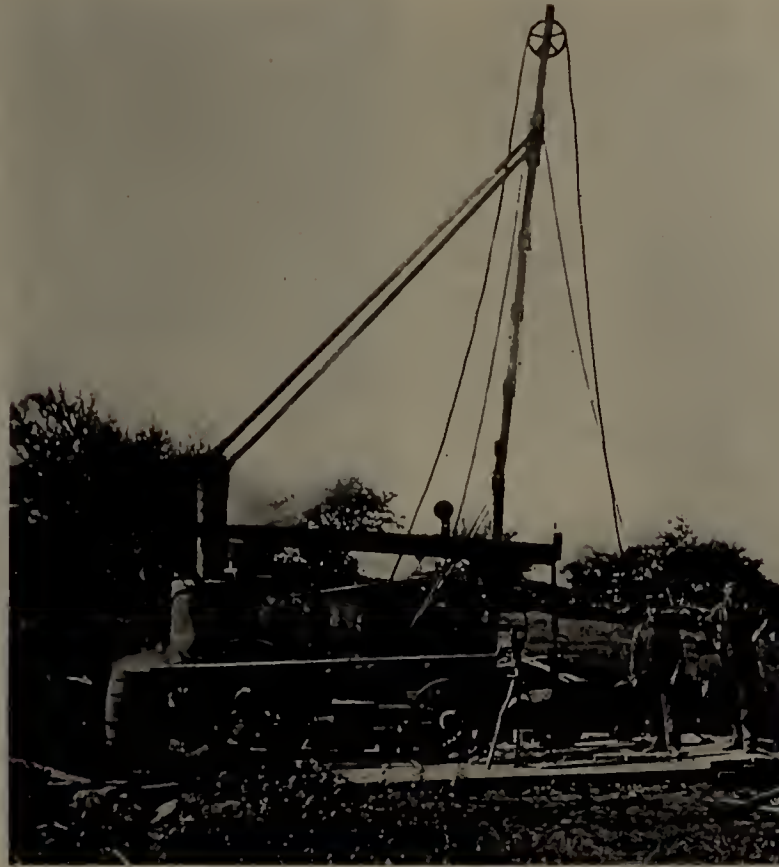
J. E. FEELEY, Artesian Well Borer, 17 Congress Street, Drilling a six-inch well for the town of Belmont, N.H.
